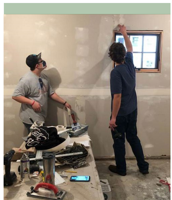
Methow Valley students learn construction trades
